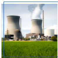
Power Generation plant
